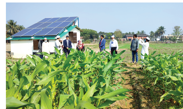
Fig. 1. Field lab installed at CA Park
